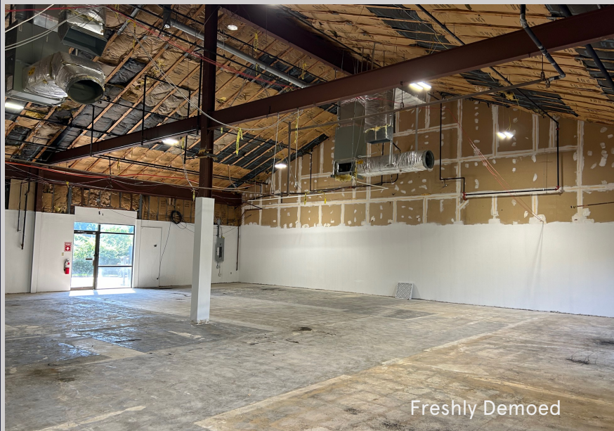
Loading Dock Interior
